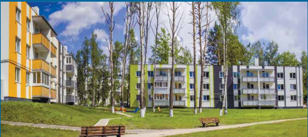
Fig. 4.33. New residential area
